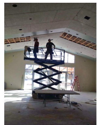
Installing acoustic panels in the Fellowship Hall
